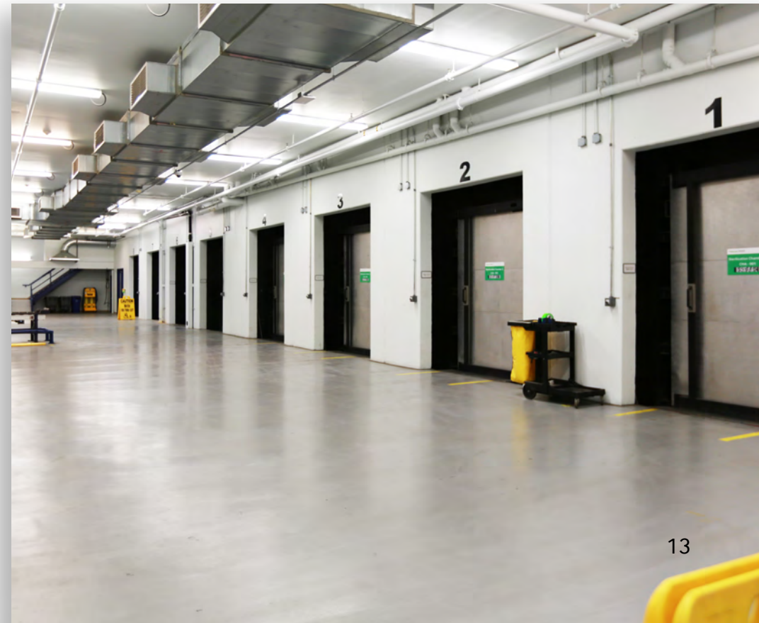
Sterilization stalls at our Lakewood, Colorado, facility
